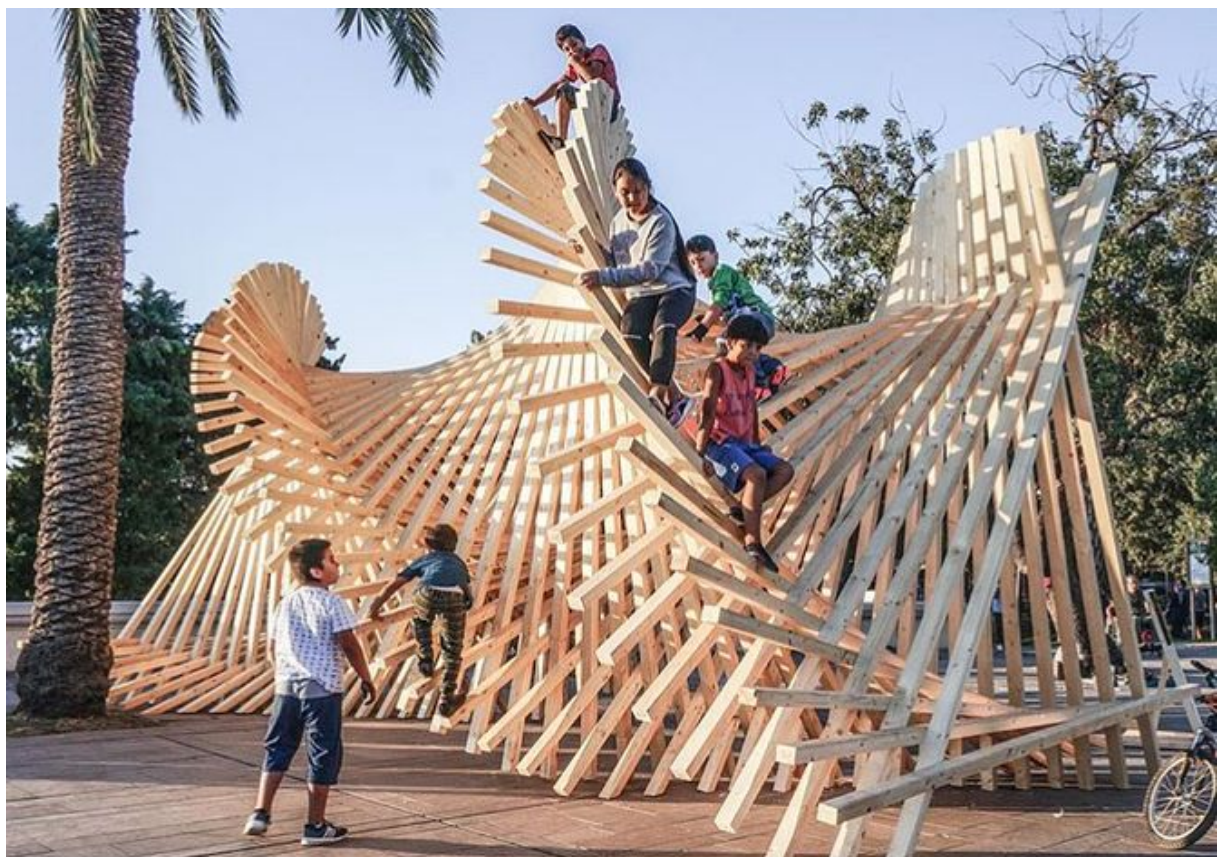
The Mediterranean Triangle : a spiral timber structure designed by MEF University students in Antalya (Turkey) for International Architecture Biennale 2017
